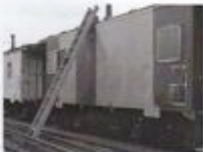
First coat of orange
